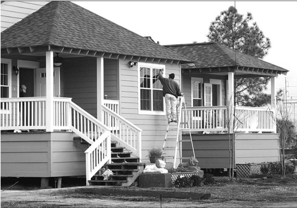
A worker adds finishing touches to completed houses at 2310 and 2314 Delery Street in the Lower 9 neighborhood, New Orleans, Louisiana. Photo credit: Marsha Cuddeback.
