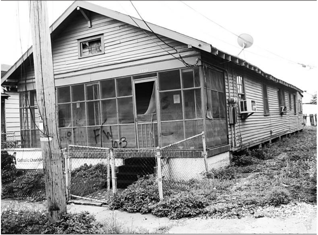
A duplex unit in the Tremé/Lafitte neighborhoods in Orleans Parish selected for reconstruction. Photo credit: James Goedert.
