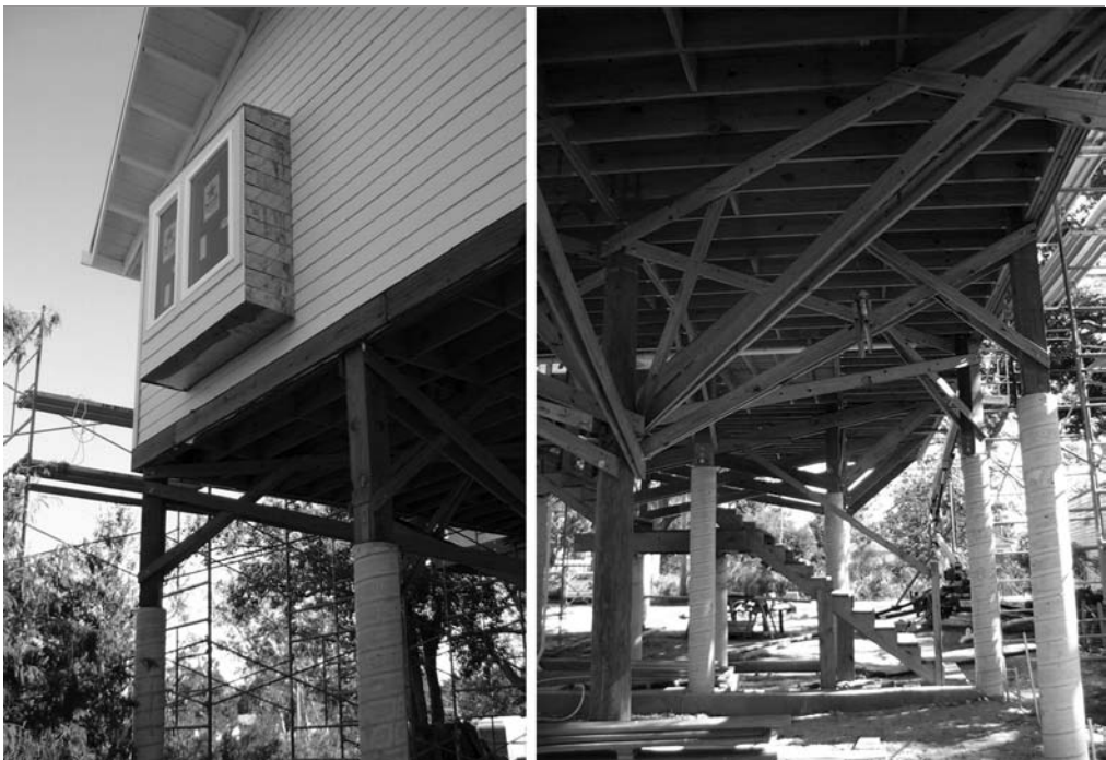
Left photo: A window box projects from the west side of the house, clad in stainless steel panels salvaged from architect Frank Gehry’s nearby art museum, which had been destroyed during Hurricane Katrina. Right photo: Bracing branches out from a center column made from a salvaged telephone pole. Photo credit: Vincent Baudoin.
