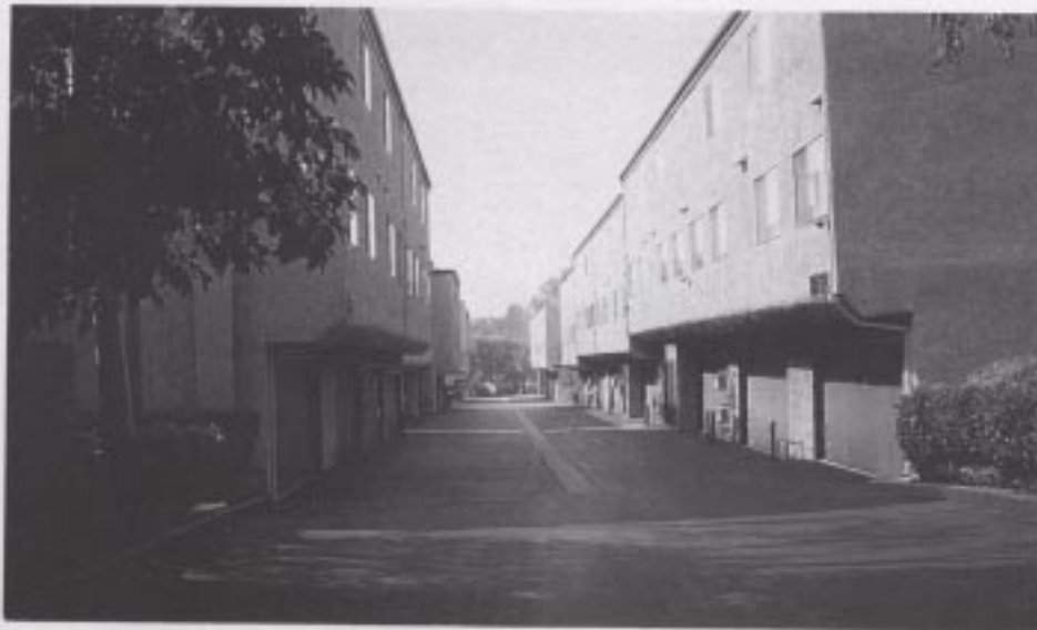
Figure 37. An example of a MFLR structure with soft-story garage construction underneath the dwelling units.
