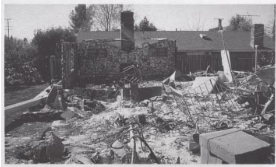
Figure 34. An example of the rare occurrence of fire damage resulting from ignited gas leaks caused by the earthquake.
