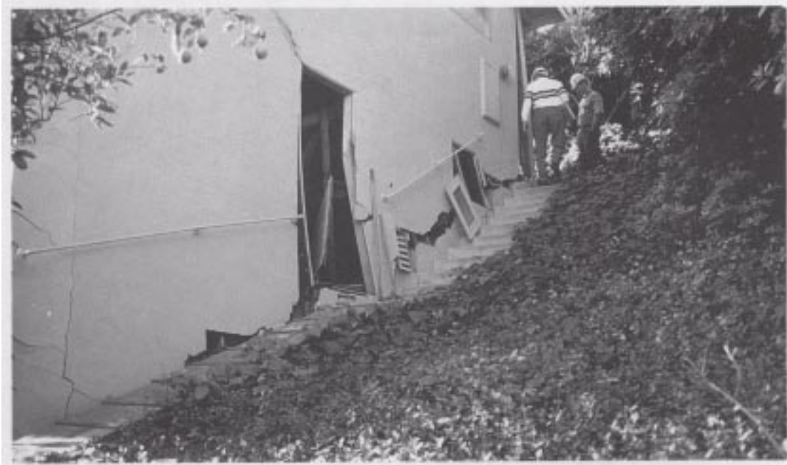
Figure 19. One example of the serious nature of foundation damage on hillside homes with a stepped foundation wall (Foundation/wall connection damage rating: HIGH)
