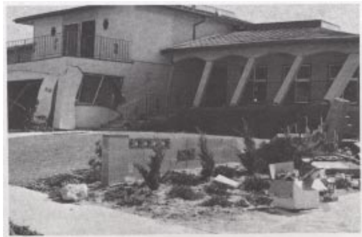
Figure 23. Photograph of the home shown in Figure 22 following the 1971 San Fernando Valley Earthquake (from “Earthquakes-Safety and Survival”, prepared by the Department of Building and Safety, City of LA, Feb. 9, 1971).
