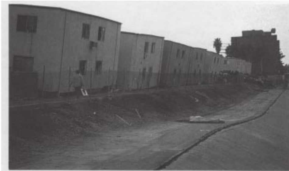
Figure 42. A soft-story collapse of MFLR buildings on Victory Boulevard Dwelling units were not located at the garage or soft-story level in this case.
