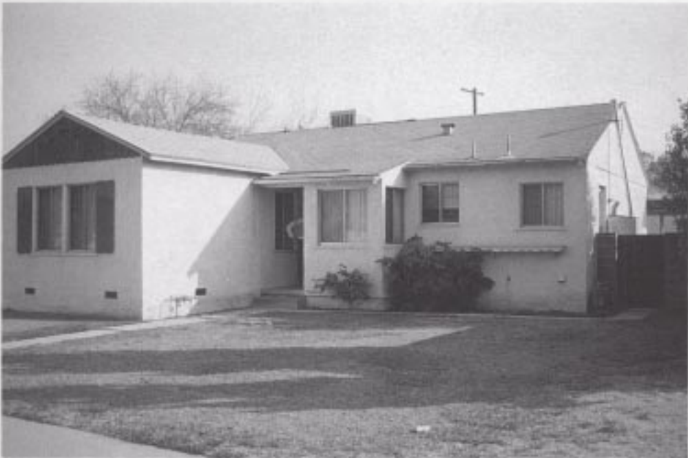
Figure 13. One of many affordable homes of "Type V" (wood-frame and stucco) construction selected for study in the SFD random survey.
