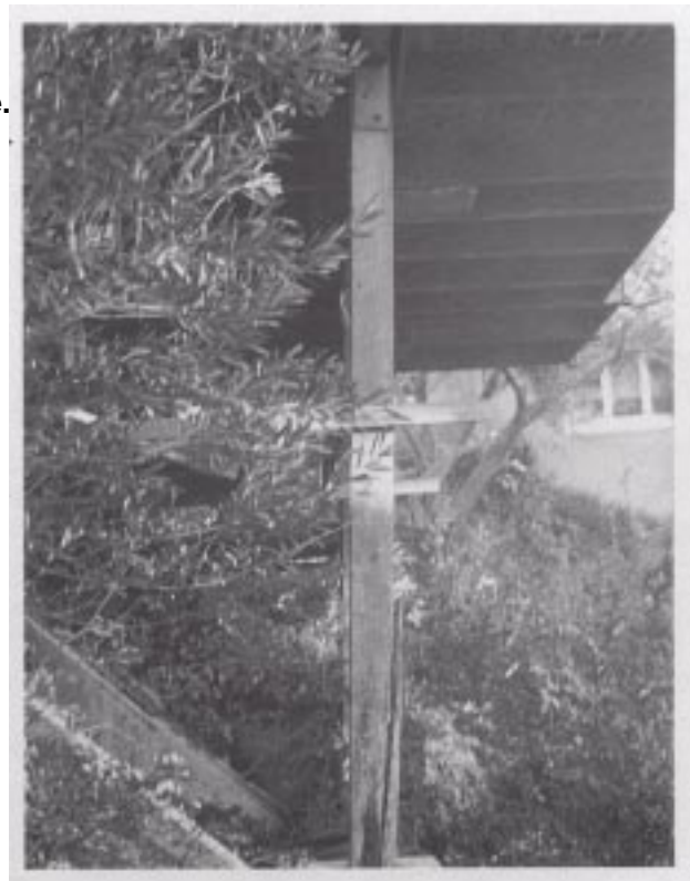
Figure 19. One example of the serious nature of foundation damage on hillside homes with a stepped foundation wall (Foundation/wall connection damage rating: HIGH)
