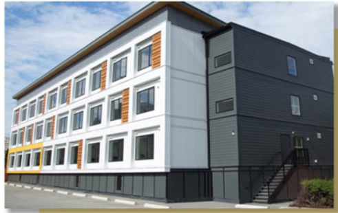
Source: NRB Modular Solutions
