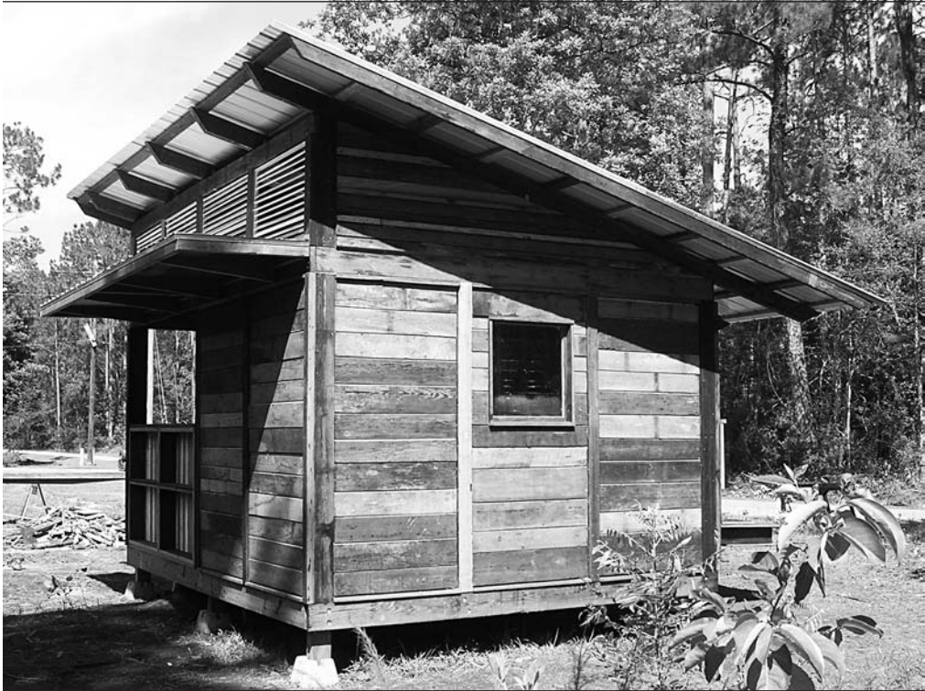
The siding, as seen on the west side of a shed built in June 2007 for Billy Ray Raines, is "barge-board" salvaged from New Orleans houses. The 2- by 6-inch posts and beams are from a deconstructed Ocean Springs, Mississippi, home. Photo credit: Brad Guy.
