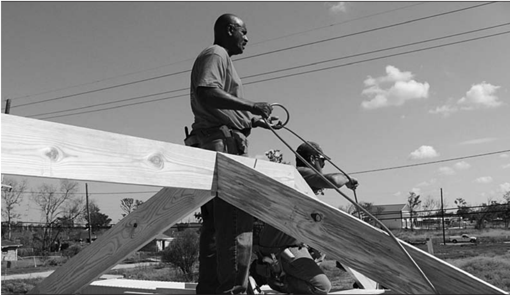
Pastor Melvin Jones, founder of Bethel Colony South, oversees the roof framing of the House at 2310 Delery Street, Lower 9 neighborhood, New Orleans. Photo credit: Marsha Cuddeback.
