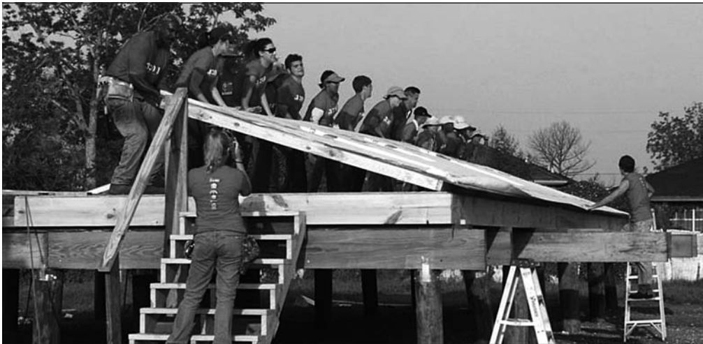
The construction team raises the first wall at 2310 Delery Street, Lower 9 neighborhood, New Orleans. Photo credit: Marsha Cuddeback.
