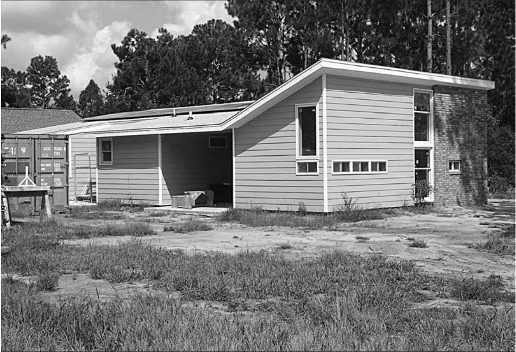
This prefabricated house in Gautier, Mississippi, includes a digital energy monitoring system that the university engineering team designed. The system collects data to chart electrical, gas, and water usage throughout the year.
