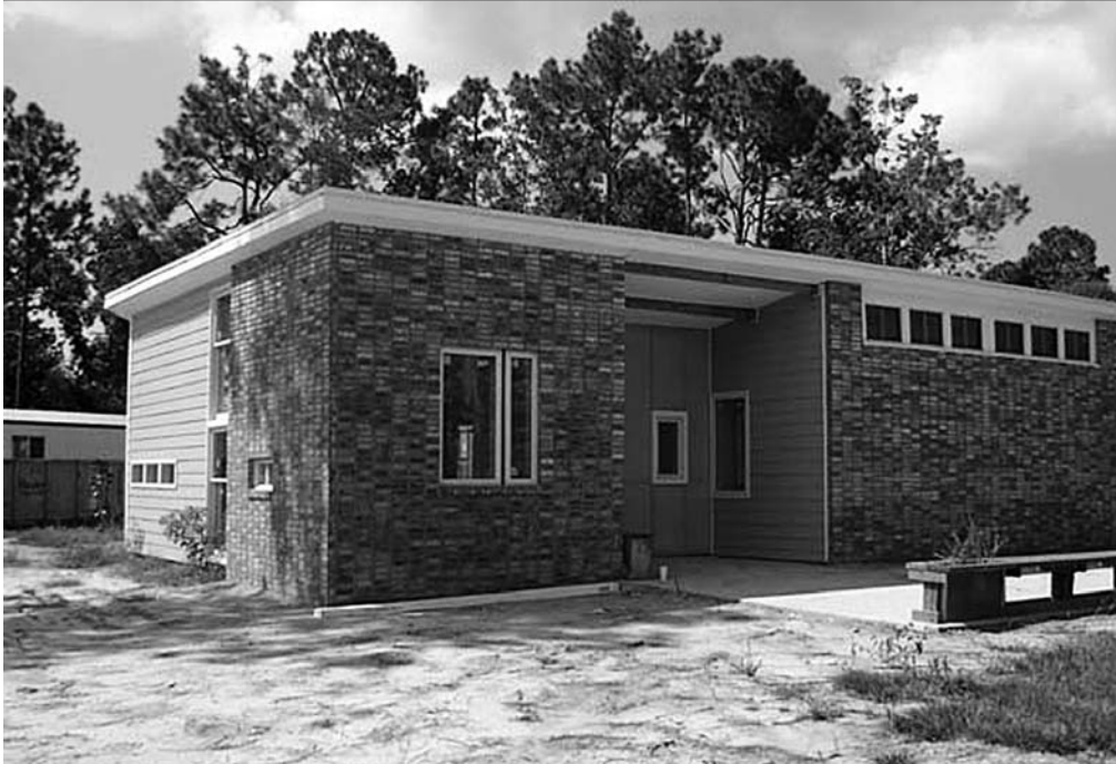
The interdisciplinary university team partnered with Habitat for Humanity International to construct this 1,087-square-foot panelized home, which was completed in Gautier, Mississippi, during the summer of 2007.
