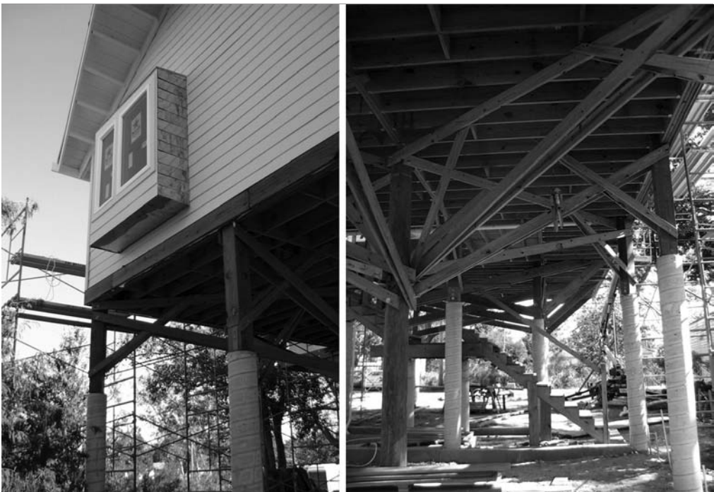
Left photo: A window box projects from the west side of the house, clad in stainless steel panels salvaged from architect Frank Gehry’s nearby art museum, which had been destroyed during Hurricane Katrina. Right photo: Bracing branches out from a center column made from a salvaged telephone pole. Photo credit: Vincent Baudoin.
