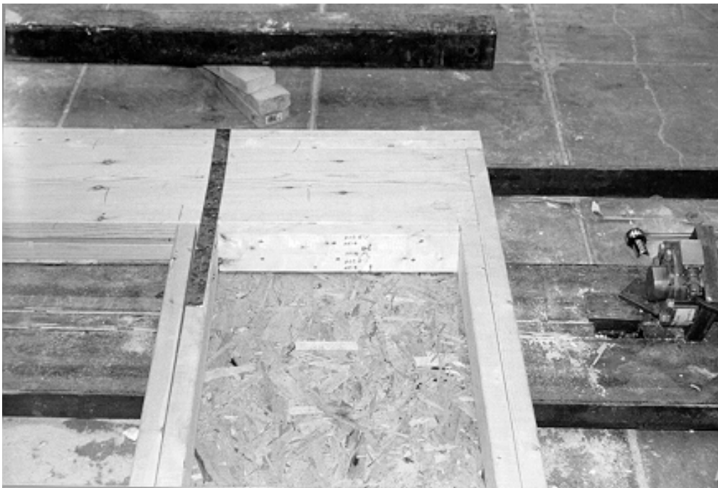
Figure 1 Alternative Framing Practices of Wall 5
