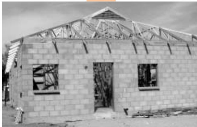
Fig. 4-16a Steel-framed metal roof, Primavera Builders, Tucson, AZ
