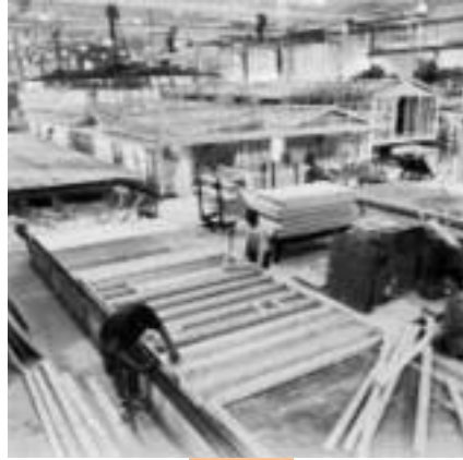
Fig. 4-6 Manufactured homes are constructed in factory-controlled conditions
