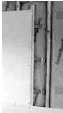
Fig. 4-41a Drywall butt joint system.
