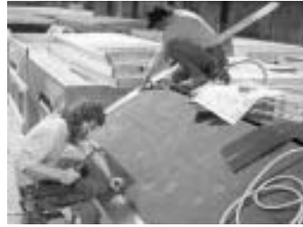
Fig. 4-4 and Fig. 4-5 Factory-built modular housing
