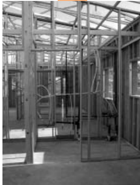
Fig. 4-16b Interior steel framing, Primavera Builders, Tucson, AZ.
