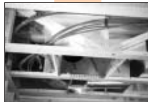
Fig. 4-33 Open-web floor joists make the installation easier.
