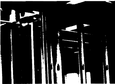
Light Gauge Steel Studs
