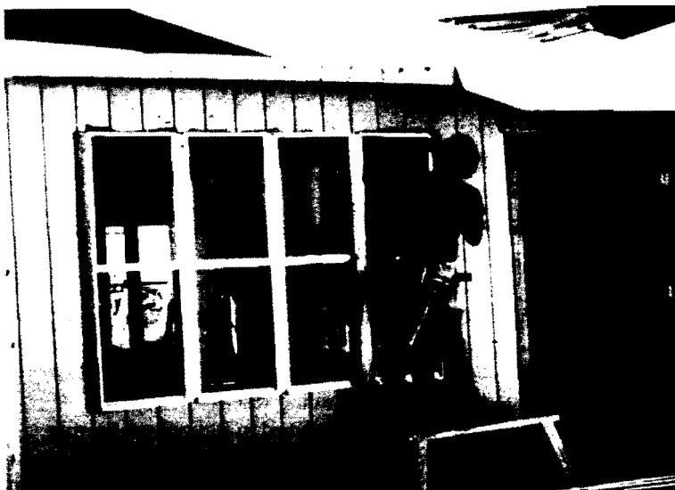
22½-Inch Wide Windows Between 24-Inch On-Center Studs
