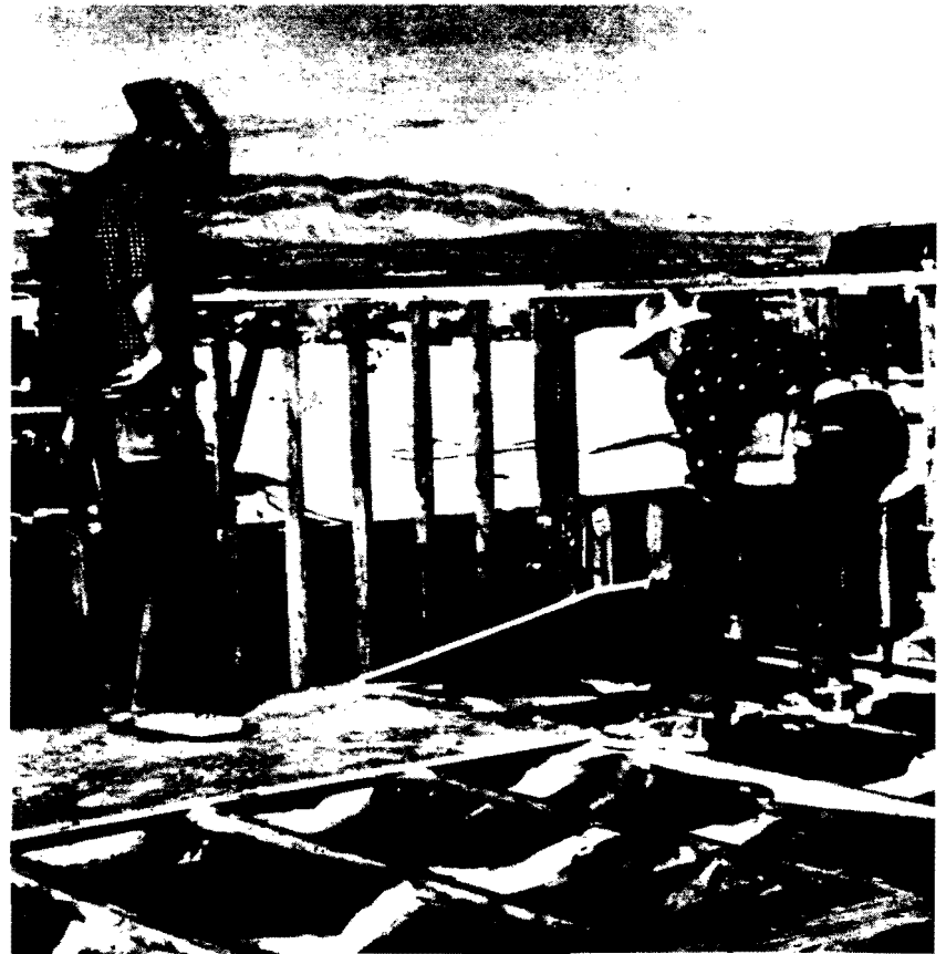
3/4-inch Tongue and Groove, Single Layer APA Sturd-I-Floor
