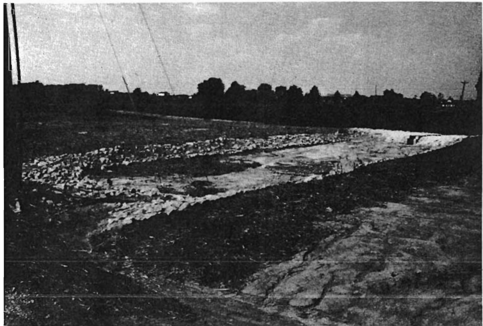
Storm water detention basin
