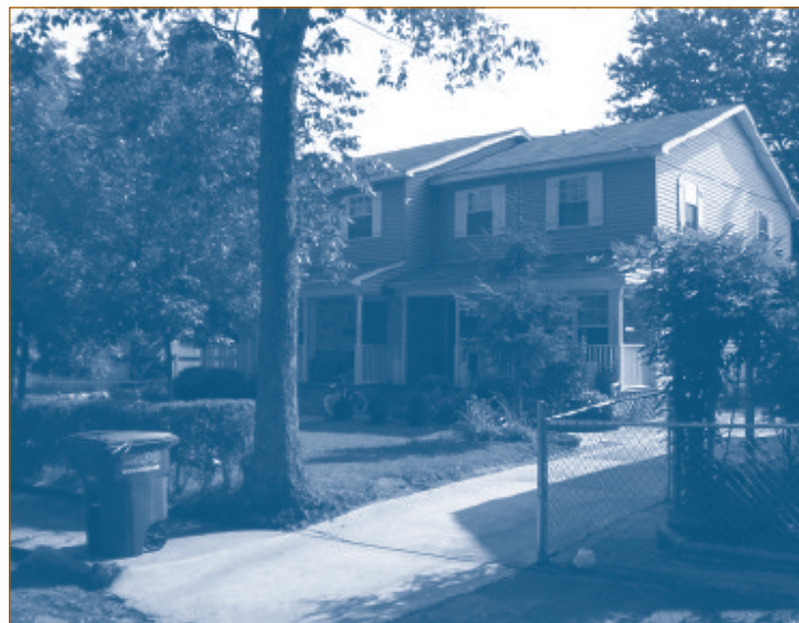
The Methodists and Mennonites (M&M) duplex built in partnership with Project Neighbors in 1999
