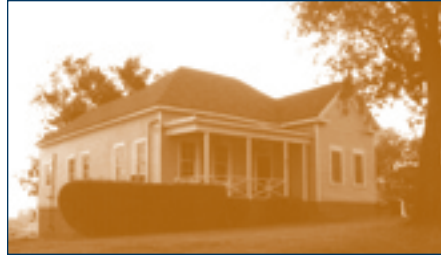
671 Ash Street after renovation
