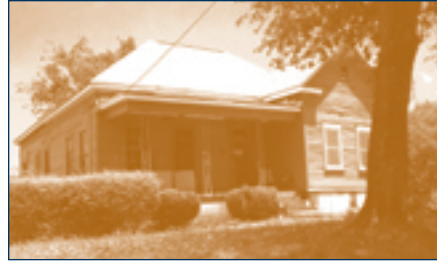
671 Ash Street before renovation
