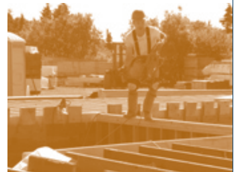
BBHA carpenter Fred Noden works on foundation system for senior housing
