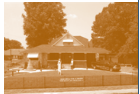
Housing project after renovation
