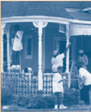
Residents help in rebuilding historic MLK neighborhood
