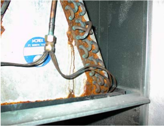
Figure 4-21. Cooling coils
