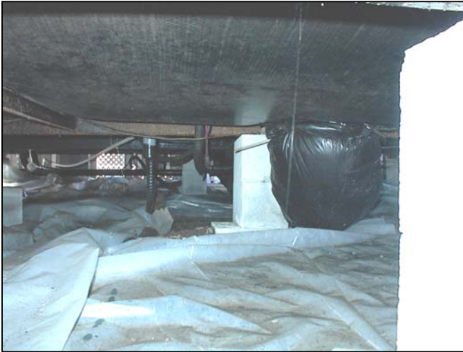
Figure 4-10. View of crawlspace showing ground cover
