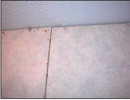
Figure 3-7. Rusty nail heads.
