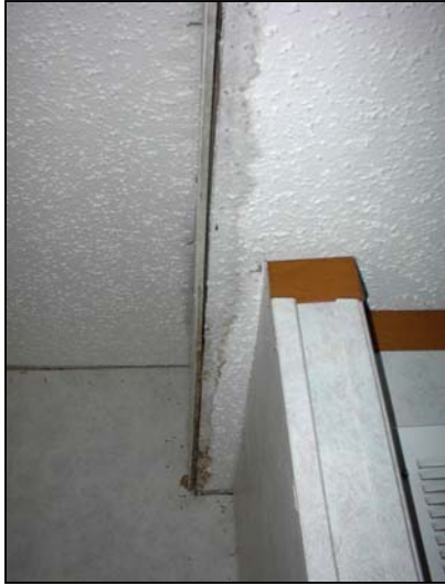
Figure 3-5. Ceiling staining.
